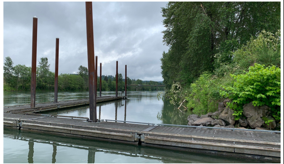
Photo 2. This photo was taken from the central dock facing south/downstream.
